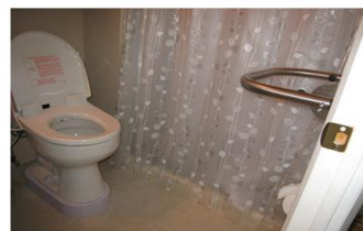
^ After: bidet and toilet riser; fold down grab bar; independent and safe toileting hygiene
