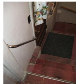
B. After: new handrails; independent in entering living area
