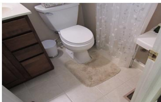
^ Before: toilet too low, unable to rise from toilet; dependent for toileting hygiene
